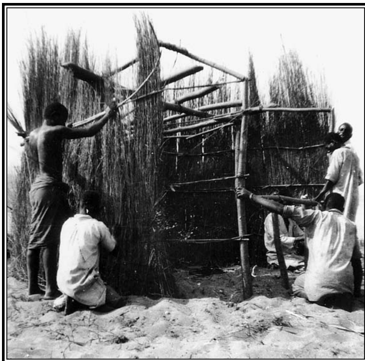
Hut Building, Kipwa, Tanganyika, 1928 This photograph, also taken by Mrs. C. Gordon, shows a reed hut in sandy soil. Note the inner construction of the dwelling.
